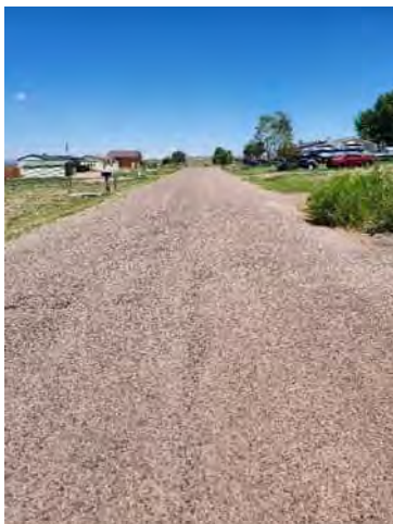
Photo 16: Highland Ave (east of curve)
