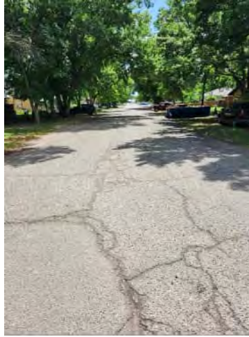
Photo 23: E 6 th St, East of N Petroleum Ave
