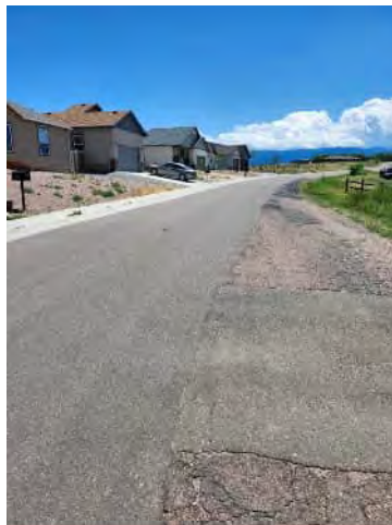
Photo 8: Arrowhead Drive (south of Highland Drive)
