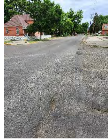
Photo 24: N Frazier Avenue, North of W 2 nd St.
