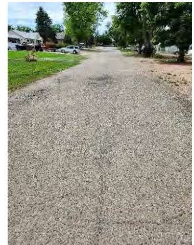
Photo 81: W 4 th St, West of Santa Fe Ave.
