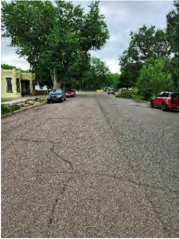
Photo 10: E 2 nd Street, East of Crawford Avenue
