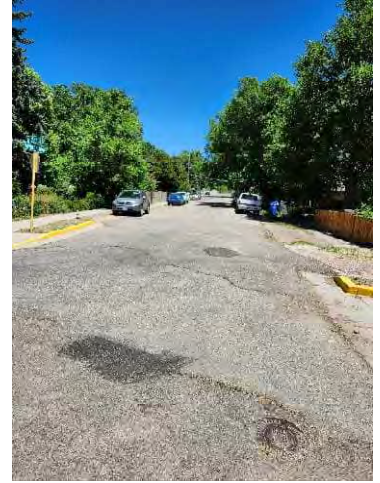
Photo 24: Hawkins Ave. north of W. 2 nd St.
