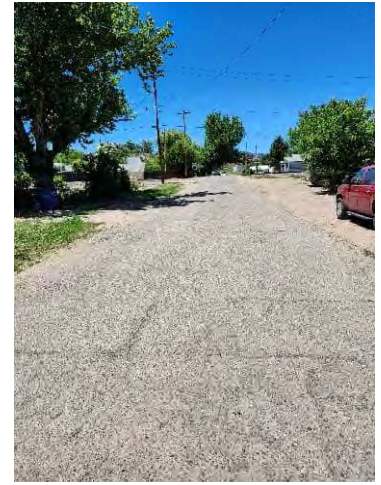
Photo 21: Houston Ave (South of W 2 nd Street)
