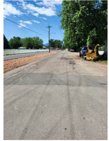
Photo 3: N Frazier Ave, at alley looking south
