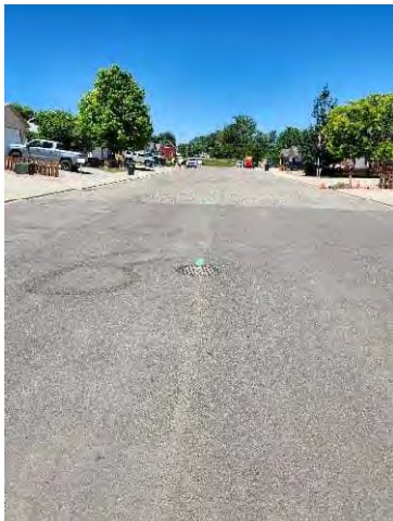
Photo 16: Rocchio Drive (looking west from end of road)
