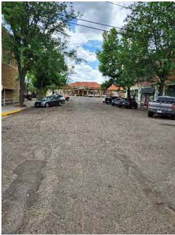
Photo 137: Railroad St, south of Front Street
