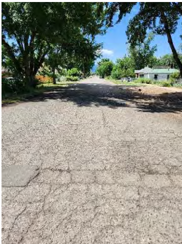
Photo 22: N Petroleum Ave south of E 6 th St.
