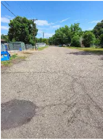
Photo 19: N Santa Fe Ave. north of W 6 th St. (Northview)
