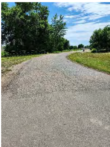
Photo 34: N McCandless Ave (at curve looking east)
