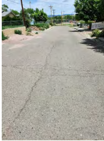
Photo 59: Gumaer Ave. S of E 5 th St Intersection
