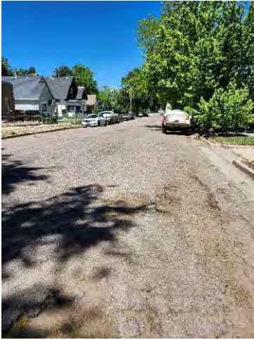
Photo 28: W 1 st Street, west of N Frazier Ave.
