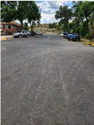
Photo 131: S Sante Fe Ave, midblock looking south
