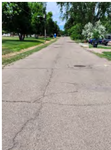
Photo 62: E 5 th St. west of Oriole Rd.
