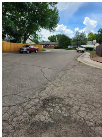
Photo 144: Loma Drive, west of Robin Rd
