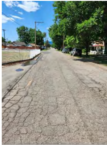
Photo 2: N Frazier Ave, north of W 5 th St. looking south
