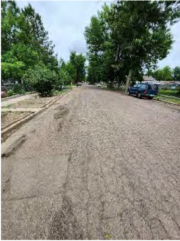
Photo 28: W 1 st Street, East of Lock Ave
