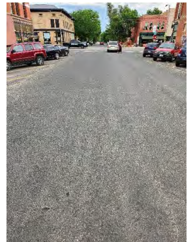
Photo 130: S Sante Fe Ave midblock looking north
