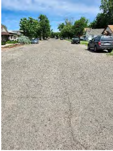
Photo 86: W 5 th St. east of N. Santa Fe Ave.
