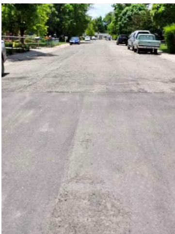
Photo 61: Oriole Rd south of E 5 th St Intersection
