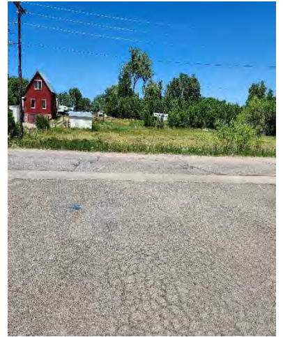
Photo 15: Rocchio Drive and Cyanide Ave. intersection
