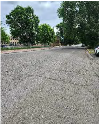
Photo 1: W 2 nd Street, East of CO-115
