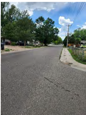
Photo 152: E 3 rd St west of Robin Rd.
