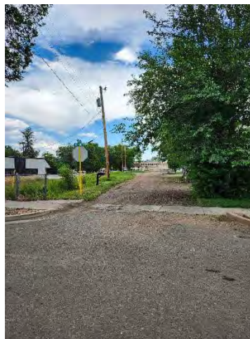
Photo 126: Grand St. east of Fremont St.
