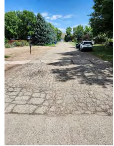
Photo 24: N Petroleum Ave, N of E 6 th St
