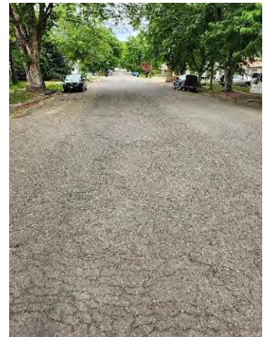
Photo 18: E 3 rd Street, West of N Pikes Peak Ave
