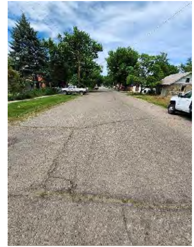
Photo 75: Petroleum Ave, North from the E 4 th St Intersection
