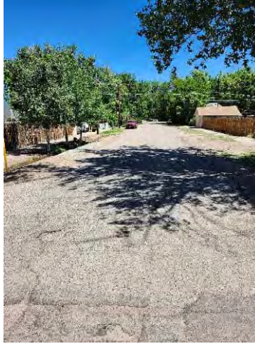
Photo 23: Houston Ave (North of W. 2 nd St.)
