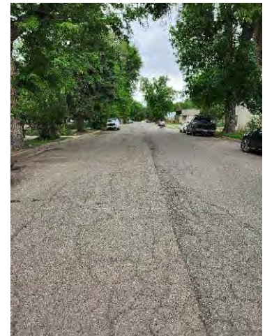
Photo 9: E 2 nd Street, East of N Robinson Ave
