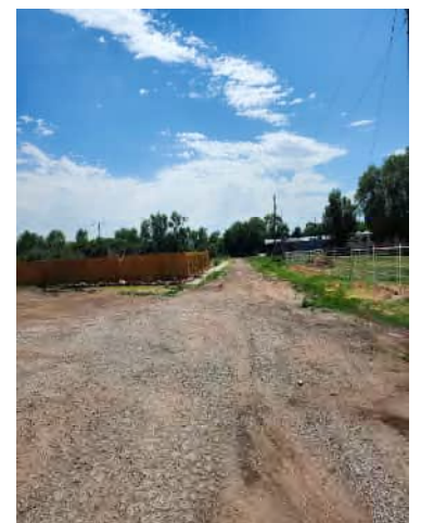
Photo 9: W 8 th St. (east of N Frazier) gravel
