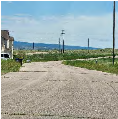
Photo 40: Sumo Ave midpoint looking northeast
