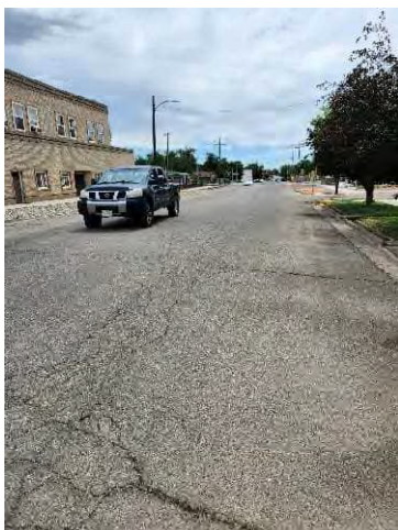
Photo 34: W Main St – west of Green St.
