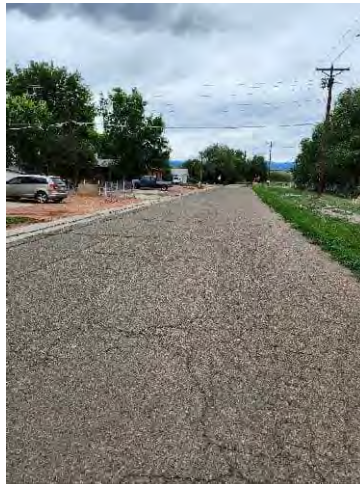
Photo 11: Florence Ave, South of E 3 rd Street
