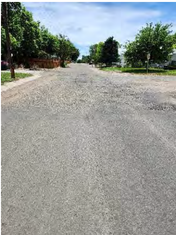
Photo 49: E 3 rd St at Sunnyside St.
