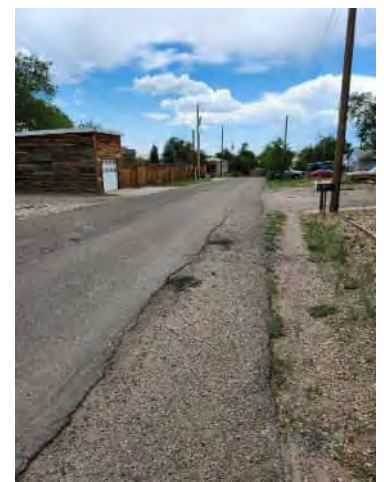
Photo 109: Granite St east of Mica St
