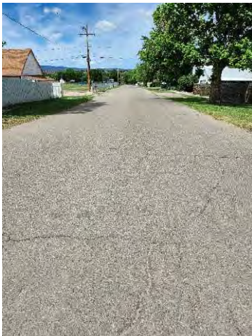
Photo 79: N Santa Fe Ave, North of W 4 th St
