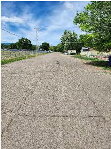
Photo 85: N Santa Fe Ave, North of W 5 th St
