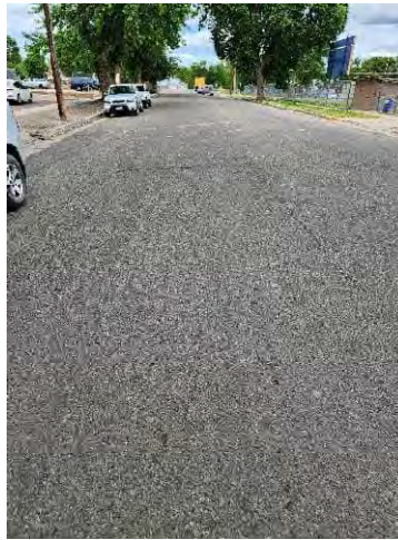
Photo 20: W 3 rd Street, West of Maple Avenue
