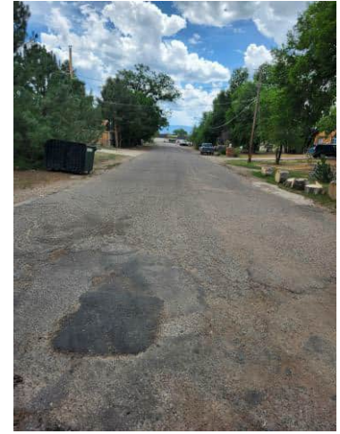
Photo 139: Sunnyside St, south of E 3 rd St.
