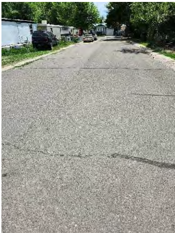
Photo 43: E 3 rd St (internal road for Alpine Village)
