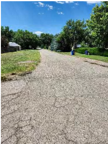
Photo 25: N Petroleum Ave south of E 7 th St (Southview)
