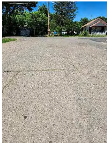
Photo 29: W 5 th St at N Frazier intersection
