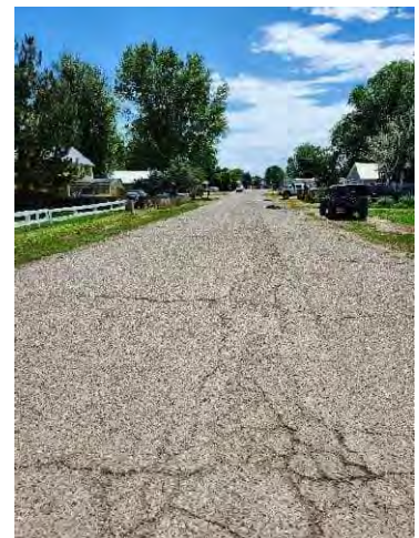
Photo 30: E 7 th St, east of Midland Ave
