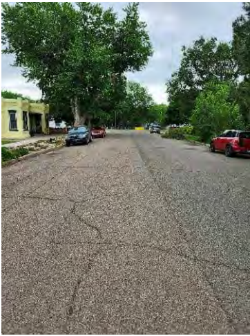
Photo 10: E 2 nd Street, East of Crawford Avenue
