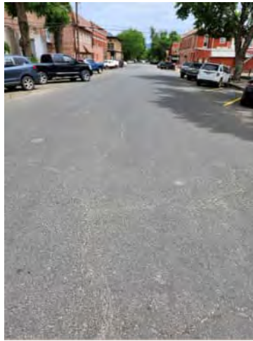
Photo 38: S Santa Fe Ave. at W Front St.
