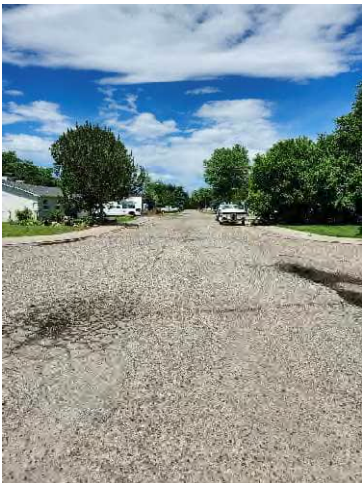
Photo 31: E 7 th St (cul-de-sac – looking west)
