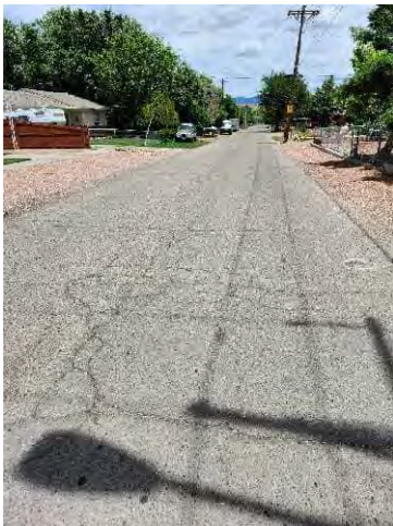
Photo 58: Gumaer Ave, N of E 5 th St
