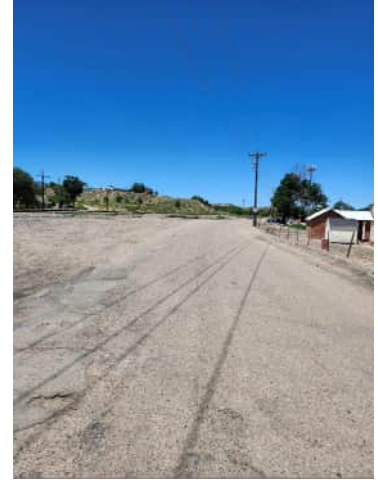
Photo 42: Railroad St, West of CO-67
