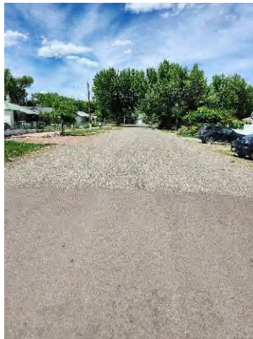
Photo 89: N Petroleum Ave (north of E 5 th St)
