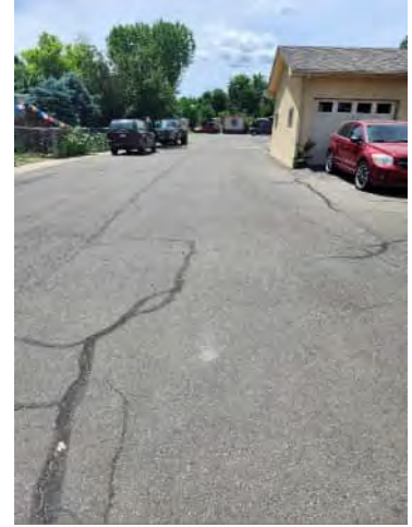
Photo 42: 722 E 3 rd St (entrance to Alpine Village mobile home park)
