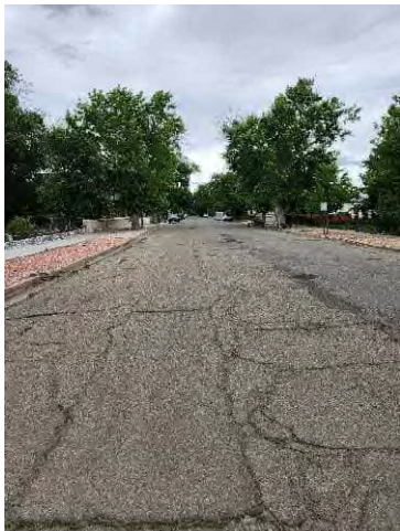
Photo 7: E 2 nd Street, East of Petroleum Ave
