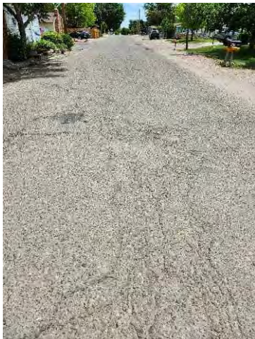
Photo 52: E 3 rd St, west of Oriole Rd
