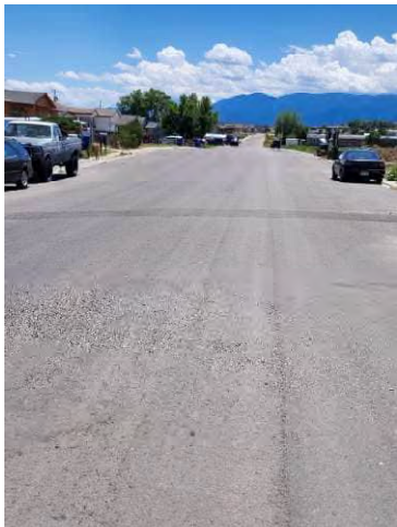
Photo 4: Arrowhead Dr (at pavement transition looking south)
