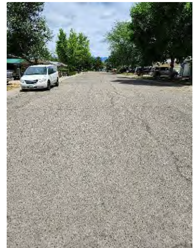
Photo 48: Meadowlark Road at E 3 rd St.
