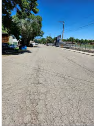
Photo 38: Church Ave north of W 3rd St.
