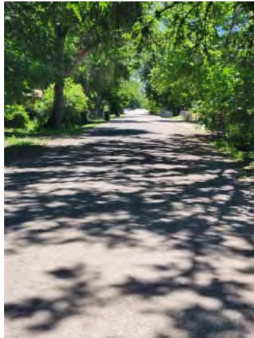
Photo 5: W 4 th St East of the City Limit
